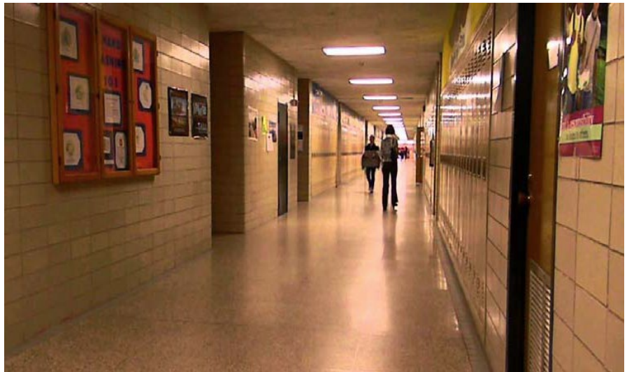
Hallway clear of obstructions and fire hazards
